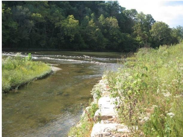
**Photo 21 .** Rock straight vane. Source: Stantec.
