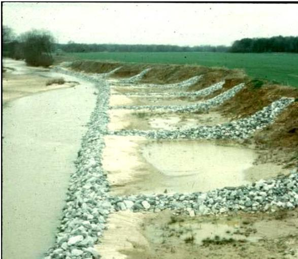
**Photo 8.** Recently constructed longitudinal peaked stone toe with tie backs; Red Banks, MS. Source: Dave Derrick
