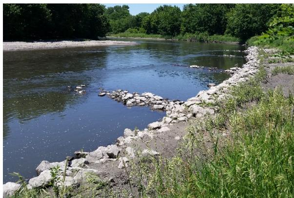
**Photo 11.** Bendway weir on Boone River after construction. Source: Iowa DNR.
