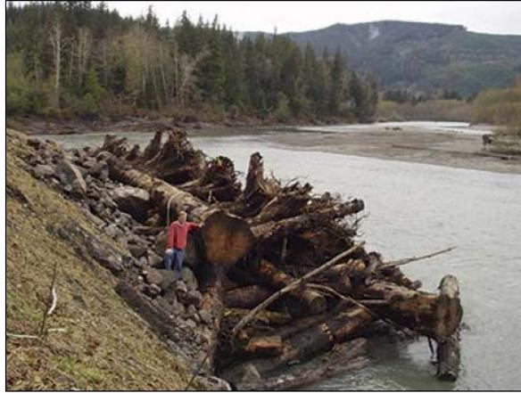
**Photo 3.** Engineered log jam on Hoh River in Washington constructed by WSDOT. Source: Herrera Environmental Consultants, Inc.
