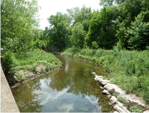
**Photo 18.** J-hook vane used to protect bank and direct stream flow through bridge infrastructure. Source: Stantec.
