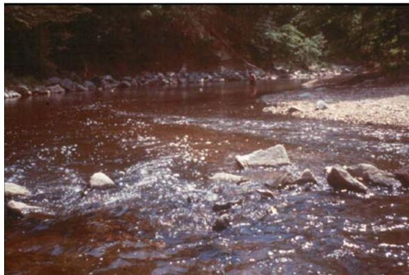
**Photo 15.** Flow over bendway weir with crest close to base flow elevation. Source: Dave Derrick.
