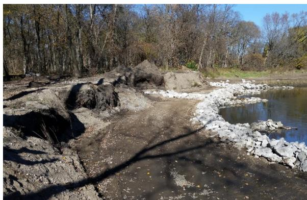
**Photo 13 .** Construction of bendway weirs on Four Mile Creek. Source: Iowa DNR.
