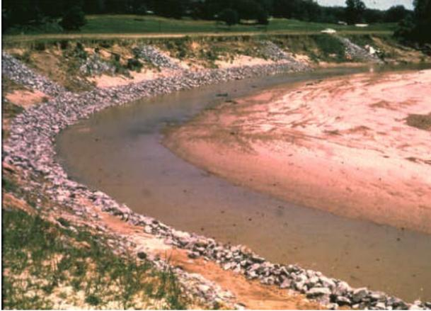
**Photo 6.** Recently constructed longitudinal peaked stone toe. Source: WES Handbook, USACE, 1997.
