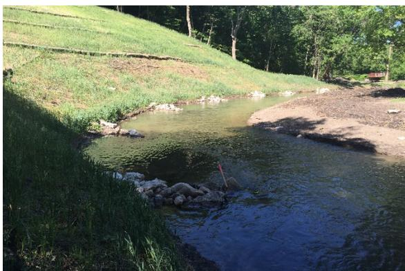
**Photo 12.** System of bendway weirs on Soldier Creek. Source: Iowa DNR.
