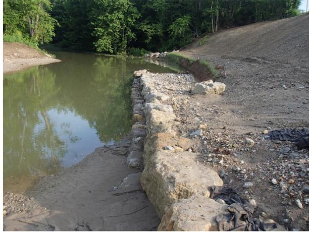
**Photo 19 .** Rock straight vane being constructed. Source: Stantec.
